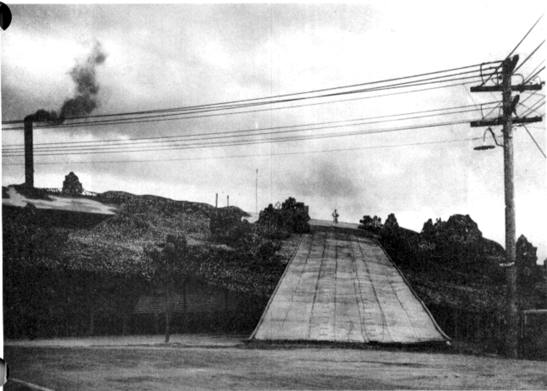
Figure 68. Ground view of a camouflaged mess hall of a munitions factory in Brisbane, Australia (1948). The false road continues on over the building and terminates logically at a route junction. This is an excellent example of camouflaging a permanent installation.
